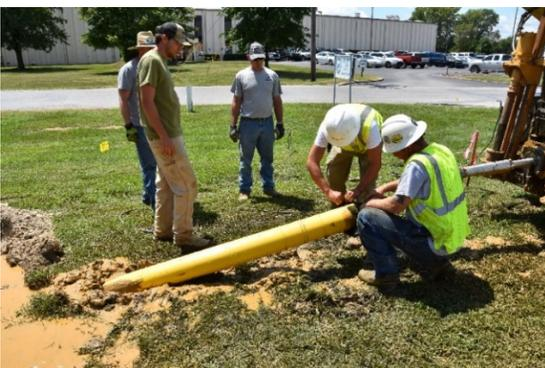
In a multi-stage project, the City of Henderson, Kentucky installed 2,720 feet of polyamide 12 (PA 12) gas pipe extruded by Teel Plastics. This marked the first PA 12 installation under the PHMSA Mega Rule effective January 2019, which allows PA 12 to be installed without a special permit.
